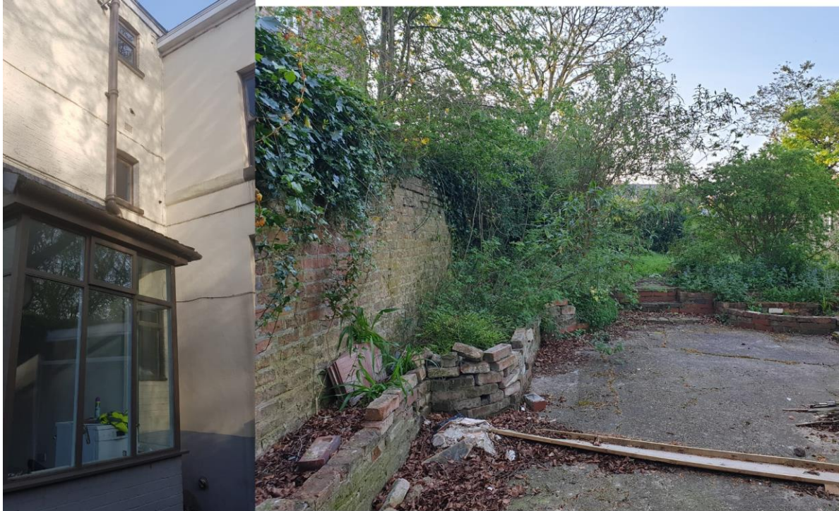
Existing bay window to the side of rear outrigger and view of boundary wall with no. 7 Norman Road
