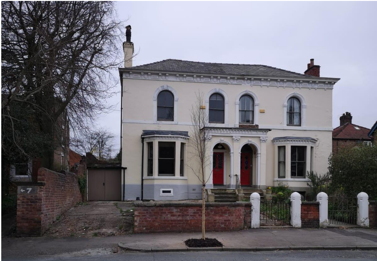
Front elevation of number 9 and 11 Norman Road (no. 9 to the left hand side)
