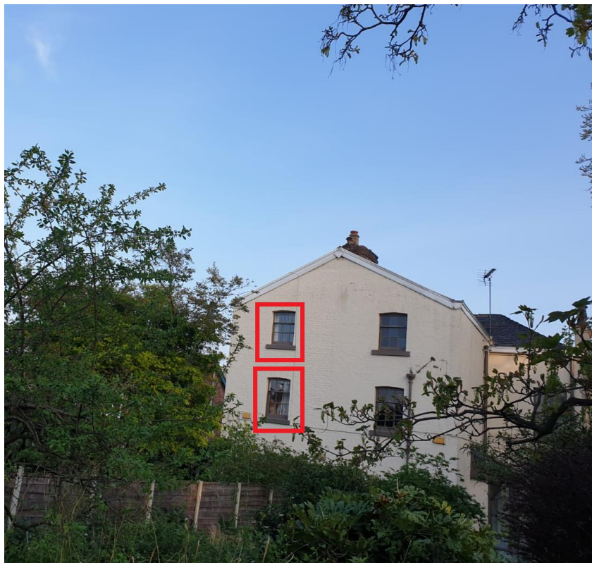
Rear view of the two storey outriggers at numbers 9 and 11 Norman Road, the rear windows of number 11 are identified edged red
